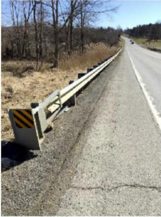
Detail 1 - Roadway Measurement Substandard* Shoulder Widths
