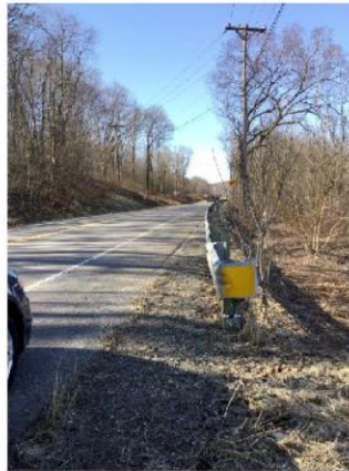
Detail 3 - Substandard* Guide Rail End Treatment Example
