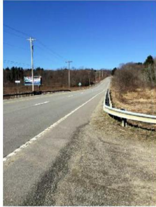
Detail 2 - Roadway Measurements Substandard* Shoulder Widths
