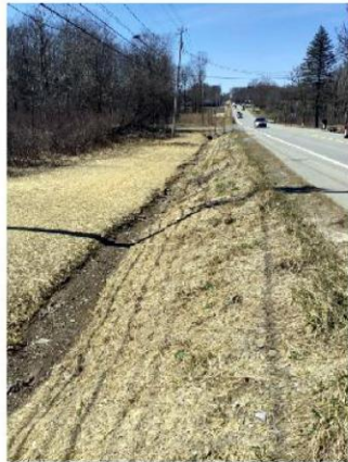
Detail 1 - Potential Need for Guide Rail Example 1
