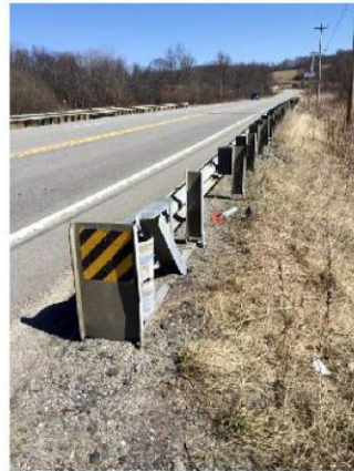
Detail 2 - Damaged Guide Rail Example
