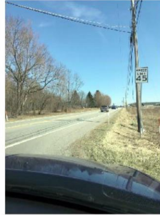
Detail 4 - Roadway Measurement Substandard* Shoulder Widths
