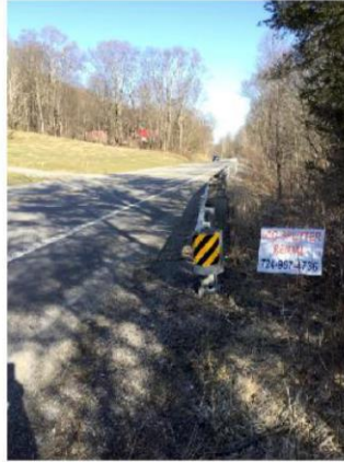
Detail 3 - Roadway Measurement Substandard* Shoulder Widths
